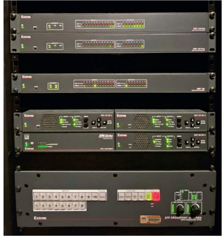
The AV system components, such as the DTP CrossPoint 108 4K IPCP MA 70 matrix switcher and the three DMP 128 audio processors, are rack-mounted within the control room.
