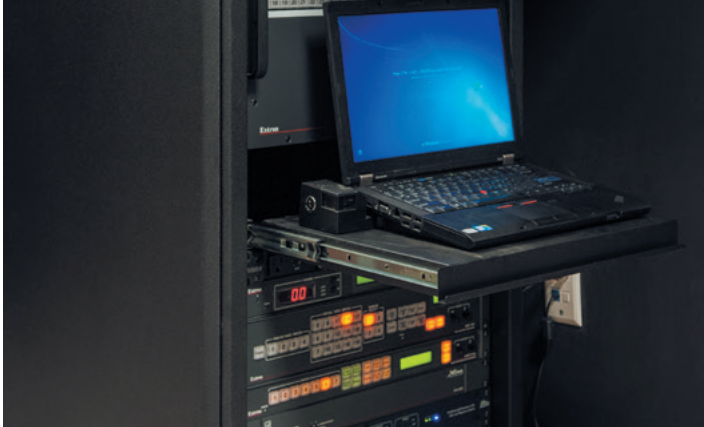
AV equipment for the Executive Conference Room is rack-mounted in a room located behind the embedded 103" plasma display.
