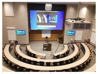
Lecture Hall viewed looking toward stage. The presenter podium is at center stage. The AV operator desk is stage left. The projector is seen in the foreground. The projection screen is flanked by two flat panel displays. A PTZ camera facing the audience is mounted to the wall at the lower right corner of the projection screen.
